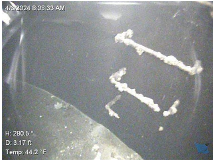
Damaged Ladder
